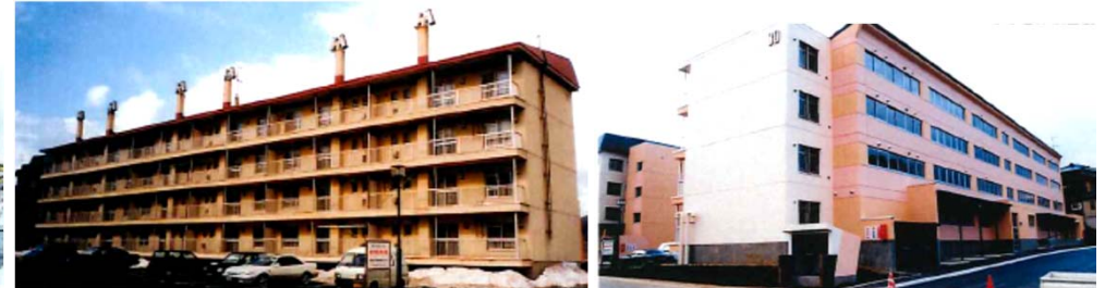
Rumoi city. Building No.30 before and after renovation
