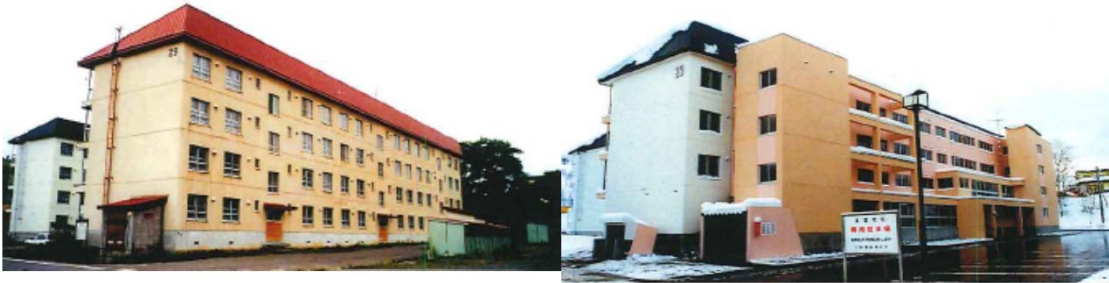
Rumoi city. Building No.29 before and after renovation
